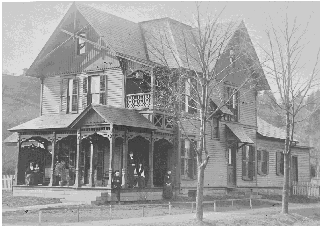
The Bryant family is pictured on their porch at the northwest corner of North Pearl and East College streets.
