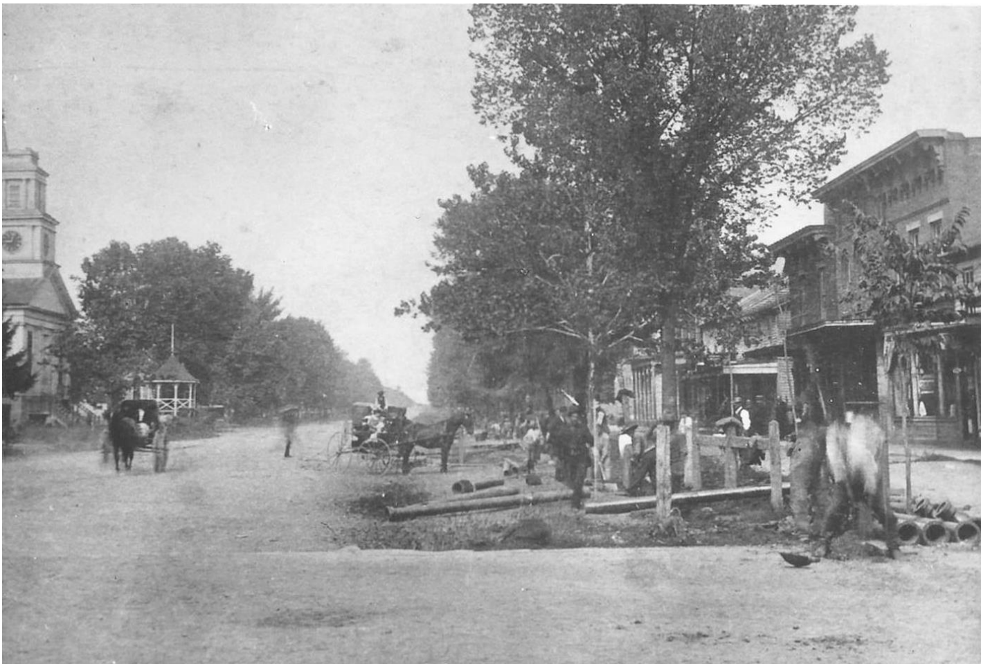
Installation of a village water system was among the achievements under Mayor “Aug” Rogers. This photo shows lines being installed on East Broadway downtown.
