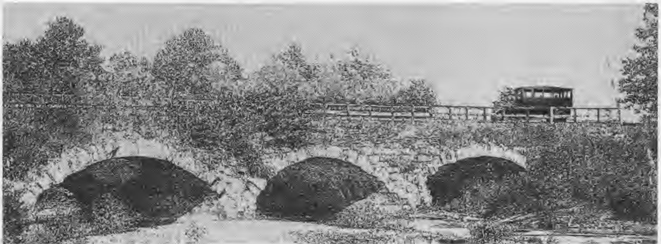
After the Interurban era was over, a bus line used the Arch. The original stonework was later faced.
