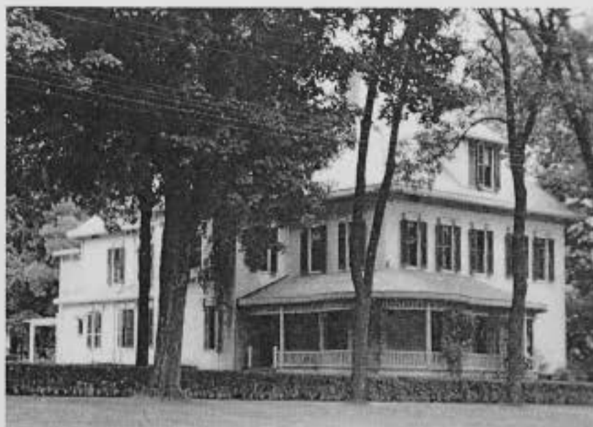
When Denison acquired it in 1935, Monomoy still sported its turn-of-the-century wrap-around porch, as it did through the 1940s. The third-floor ballroom, also turn-of-the-century, dramatically changed the earlier proportions of the house.
