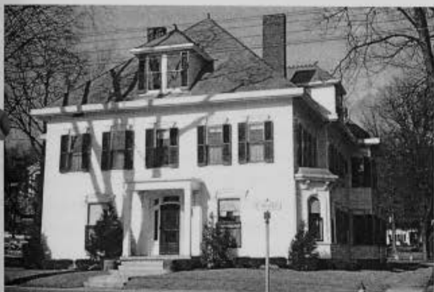
The large porch was removed and replaced in the early 1950s with a simple square portico when it became cooperative housing for freshman women at Denison.
