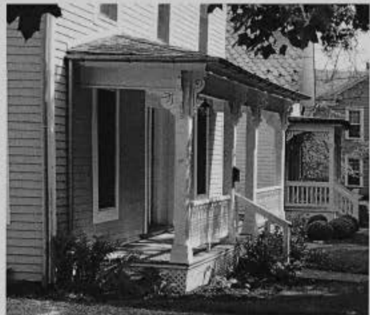
Porches were often later additions to Granville houses of all styles, creating outdoor spaces for neighborly interactions in a community where the sidewalks are still well used.
