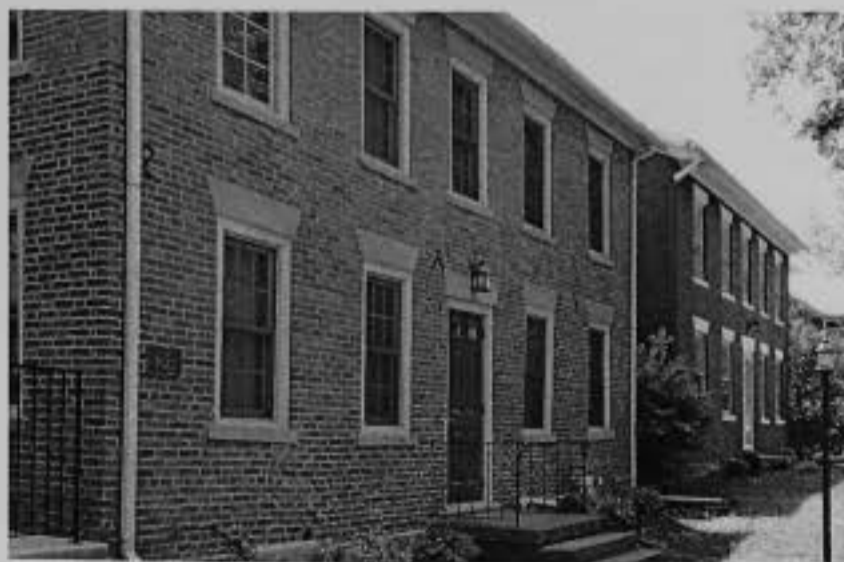
This pair of nearly identical brick homes was built by Allen Sinnett, a local blacksmith, in 1822 and 1823. They reflect a simple variation of the vernacular Federal style of the time.
