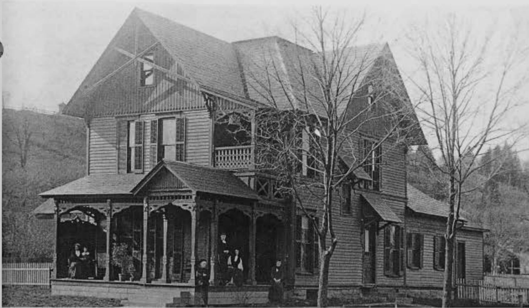
Pen Coed, still thriving at the corner of College and North Pearl streets, is a rare example of the Stick style in Granville.
