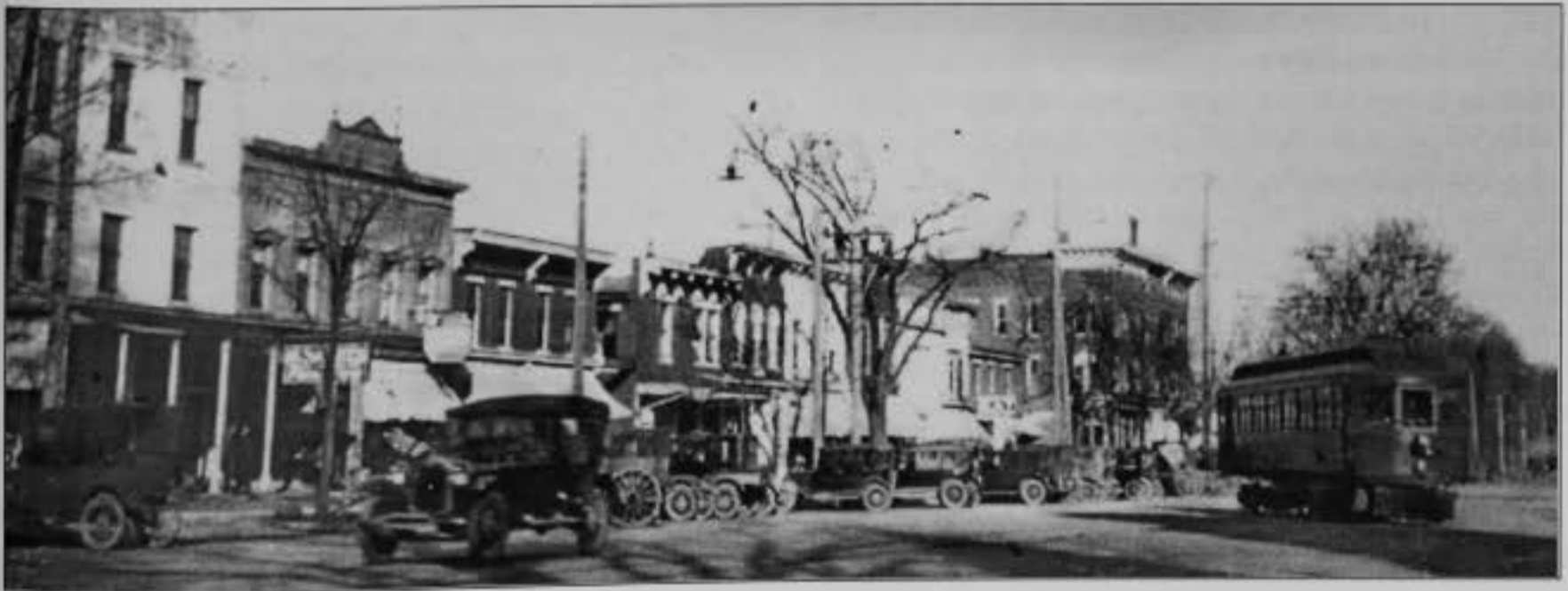
In its last decade before its 1925 closing, the Interurban turns from East Broadway into the station, which is today's Granville Historical Society Museum.
