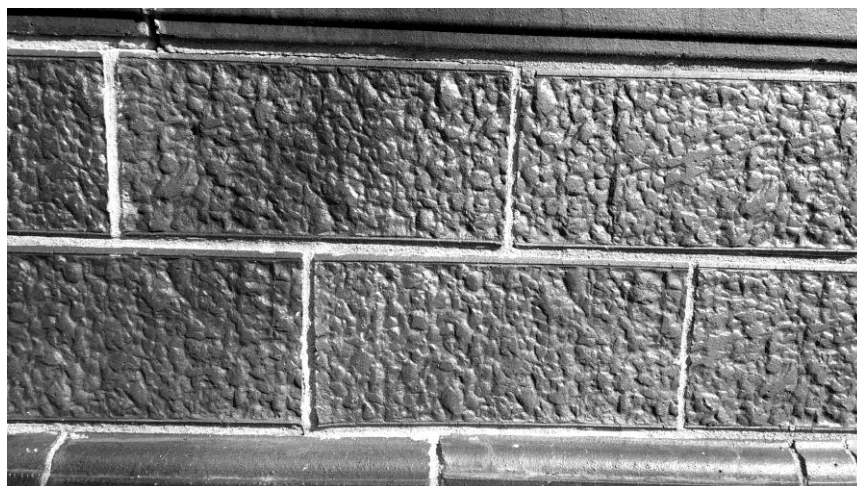
Foundations on homes around Granville often have a fake stone block on the outside (top) and glazed block on the inside (directly above).
