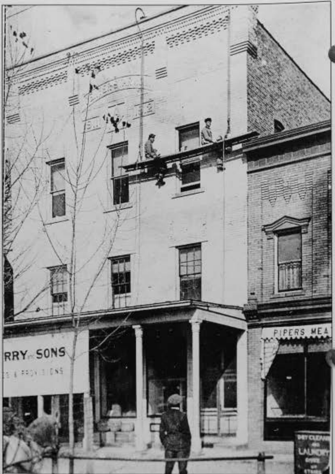
Guy Rodes and James Clark working on the addition to the building (photo courtesy of Virginia Williams)
