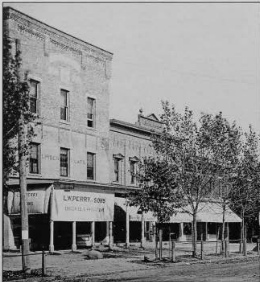
On the far left is the building after the 1912 addition of the third floor, and during the grocery proprietorship of L.W. Perry & Sons. This photo was taken before stucco and paint were used to harmonize the older part of the building with the addition. (Photo courtesy of the Granville Historical Society)
