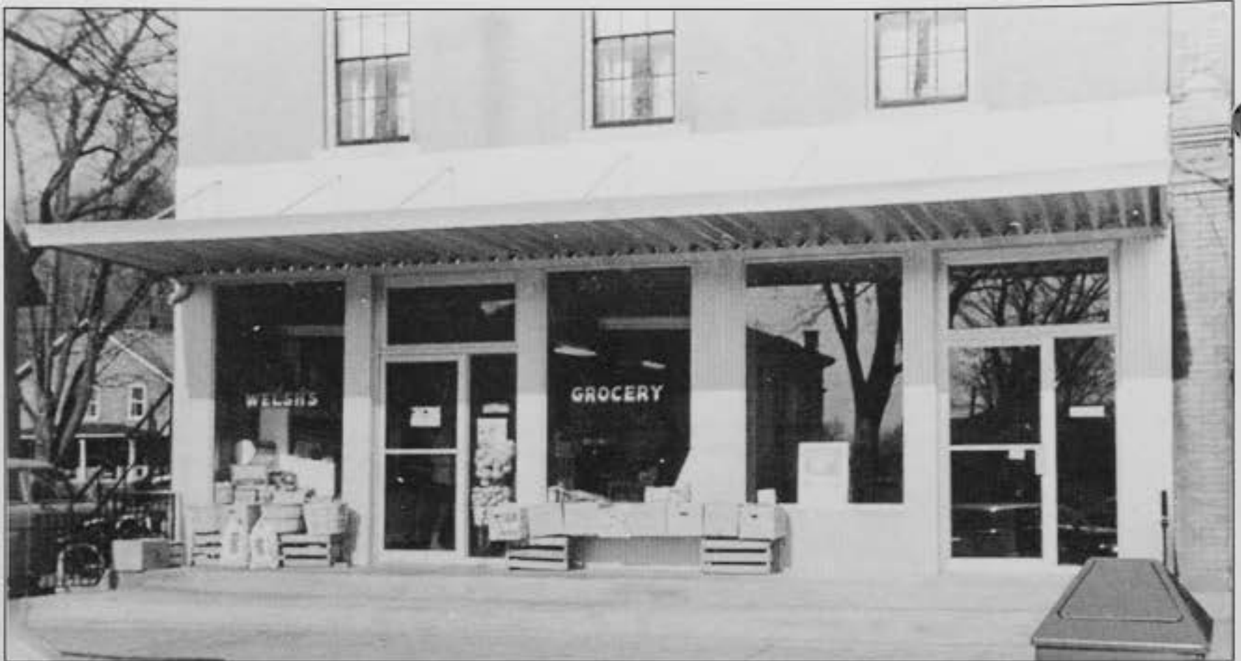
Carl Welsh's Grocery following the modernization of the façade. This photo shows the partition of the storefront into two shops, the larger on the west. The small east-side shop was used by James Remmele for his financial services office during part of the time that Welsh's Grocery was on the west side. (Photo courtesy of Jennifer Welsh and Family)
